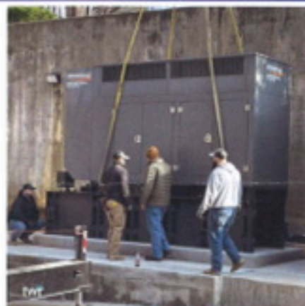
Installation team works with TWR staff to install a new generator at the int'l corp. office
